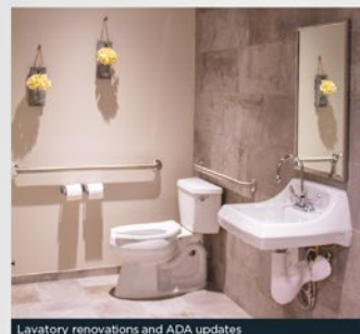
Lavatory renovations and ADA updates
