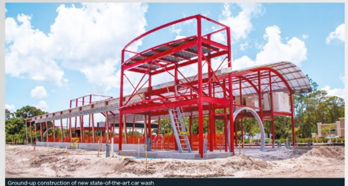
Ground-up construction of new state-of-the-art car wash
